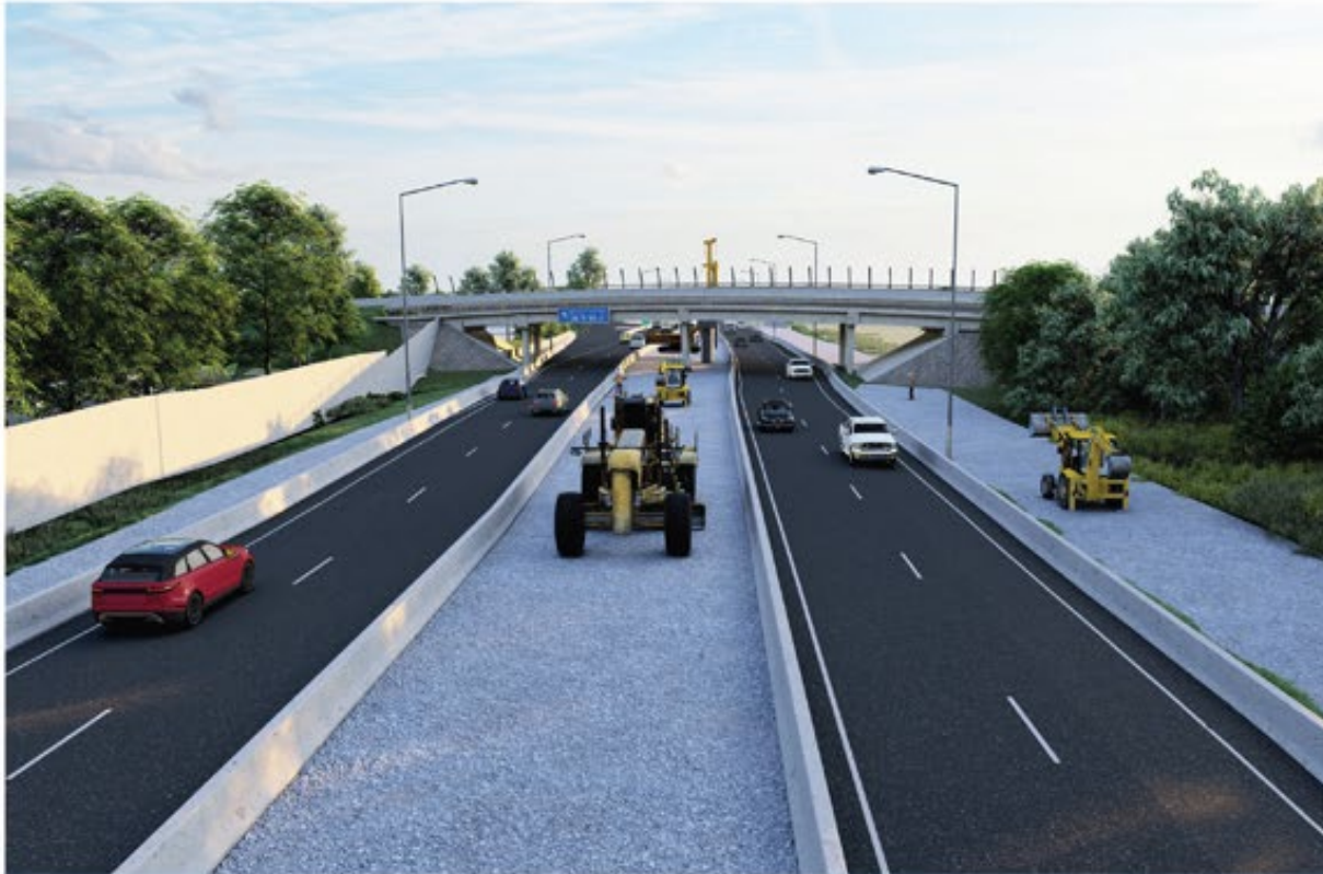
PHASE 1 commenced in April 2021 and is in progress.
