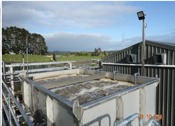
Membrane live air scour testing
