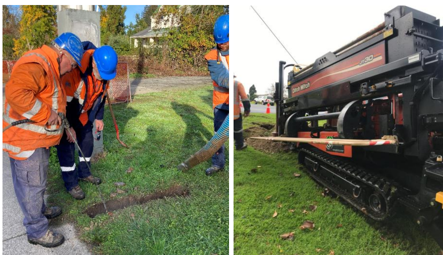
Watermain Renewals: service location and pipe drilling works
