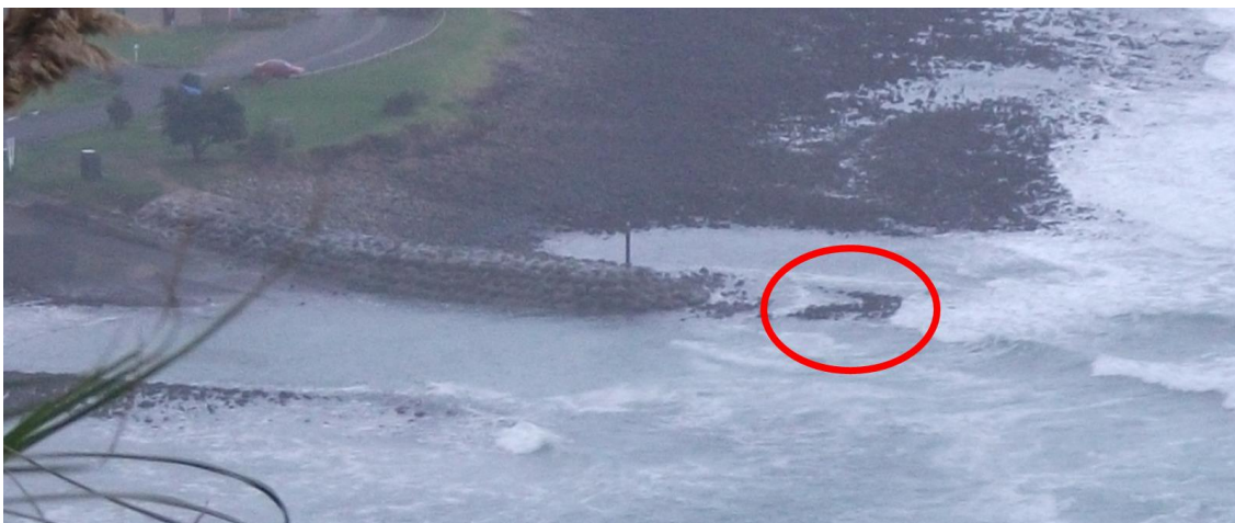
Figure 12: Rock mound beyond the tip of the breakwater highlighted by the red circle. (Source: WDC).
