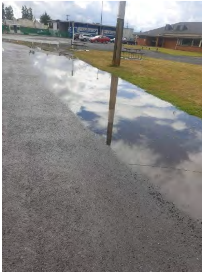
Photo of ponding whenever it rains
