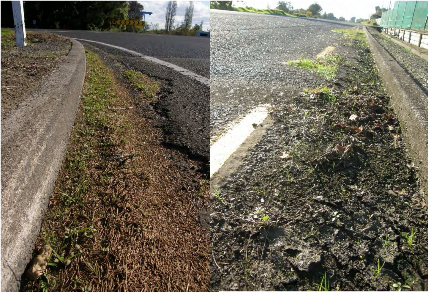
Current state of Ohinewai gutters.
