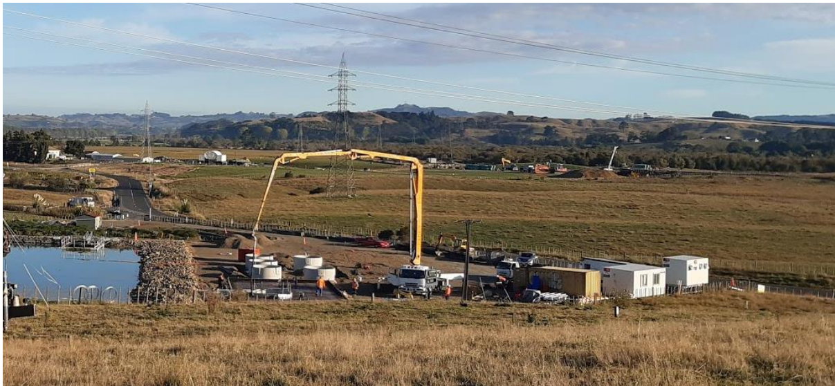
Meremere WWTP – New Inlet PS slab construction
