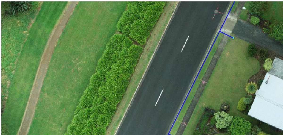
Waipa Esplanade Watermain Renewal – Completed Utility Mapping and Route Planning
