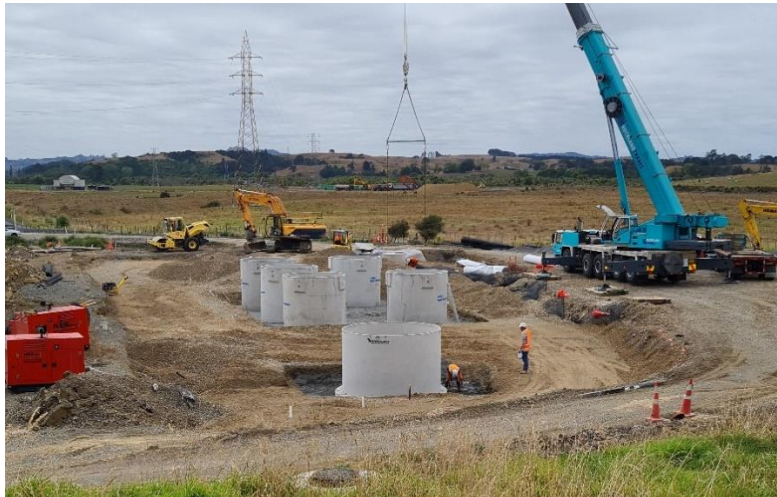
Meremere WWTP – New Inlet PS and biological process tanks
