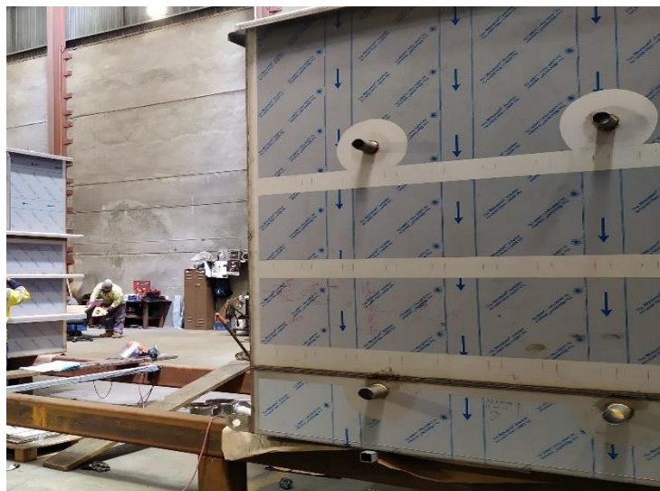
Meremere WWTP – New MBR tanks
