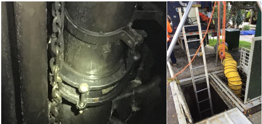
Marine Parade PS Gibault repair works
