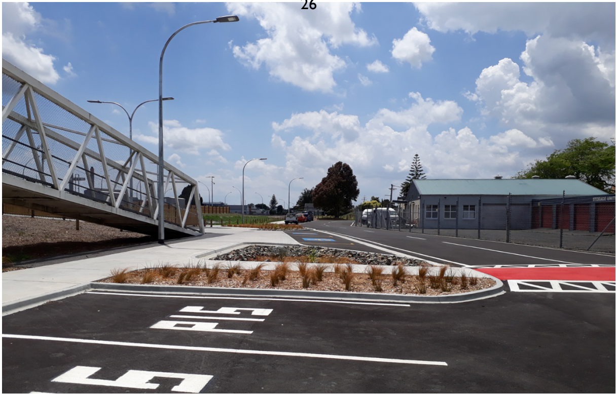
Road marking is complete.
