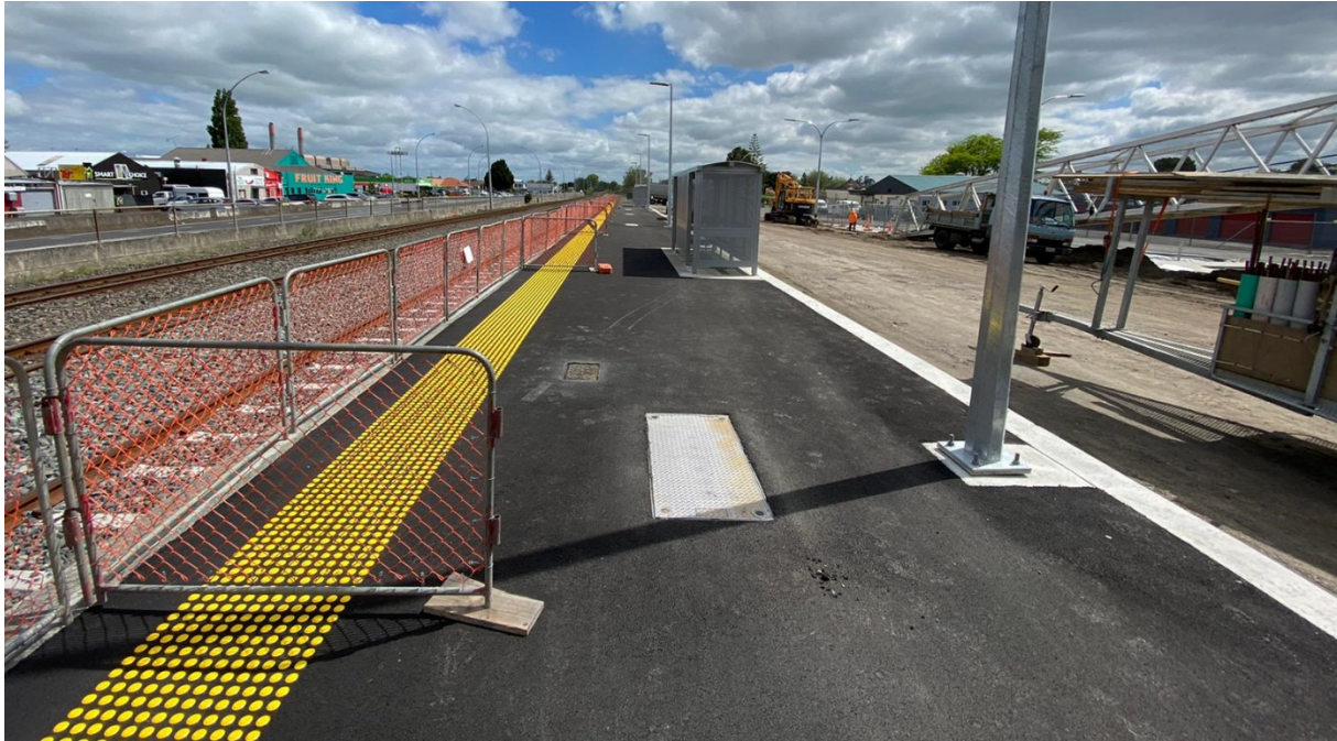
Completed railway platform
