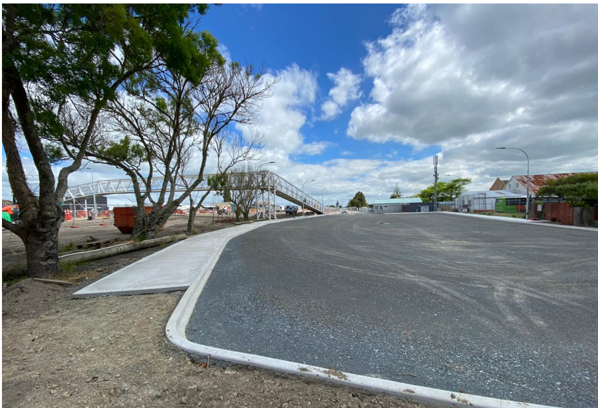
Park and Ride pavement nearing completion
