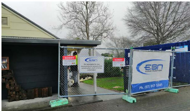
Pokeno Toilets closed for refurbishment
