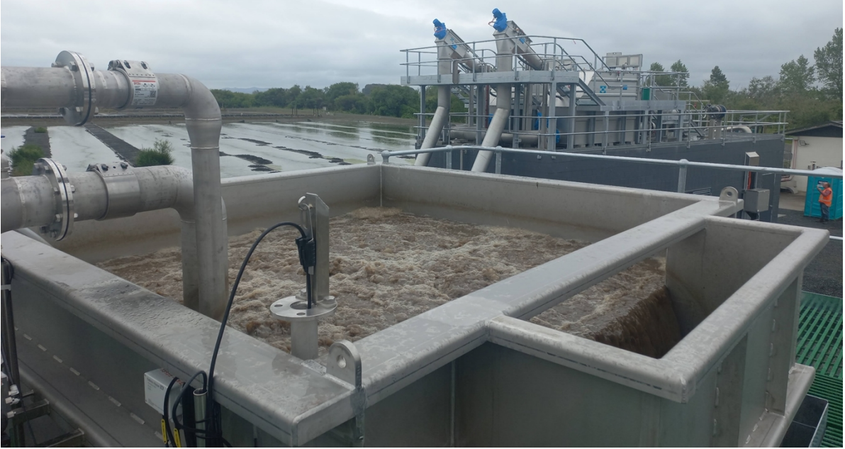
Te Kauwhata WWTP - New MBR Tank (above) New Treatment Plant receiving flow (below)
