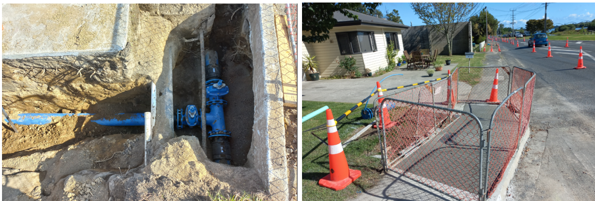
Huntly – The watermain replacement on Riverview Road is now complete.
