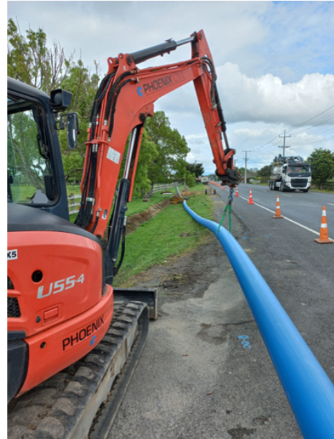
Morrinsville Road (SH26) – Pipeline installation
